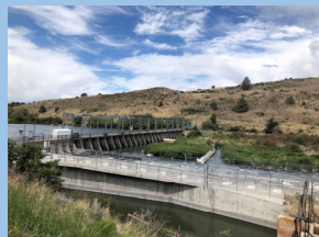
Link River Dam fish ladder
