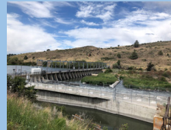
Outlet of Upper Klamath Lake/Link River Dam
